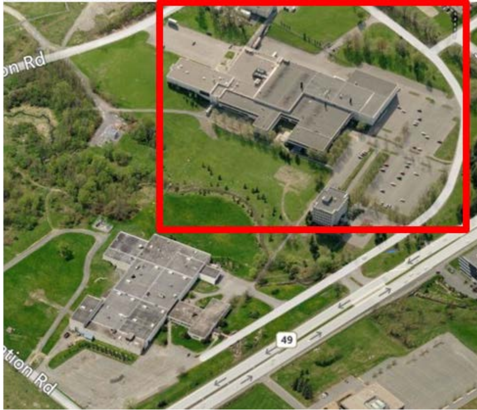
Figure 9-1: Aerial view of Nordion, Ottawa, ON
