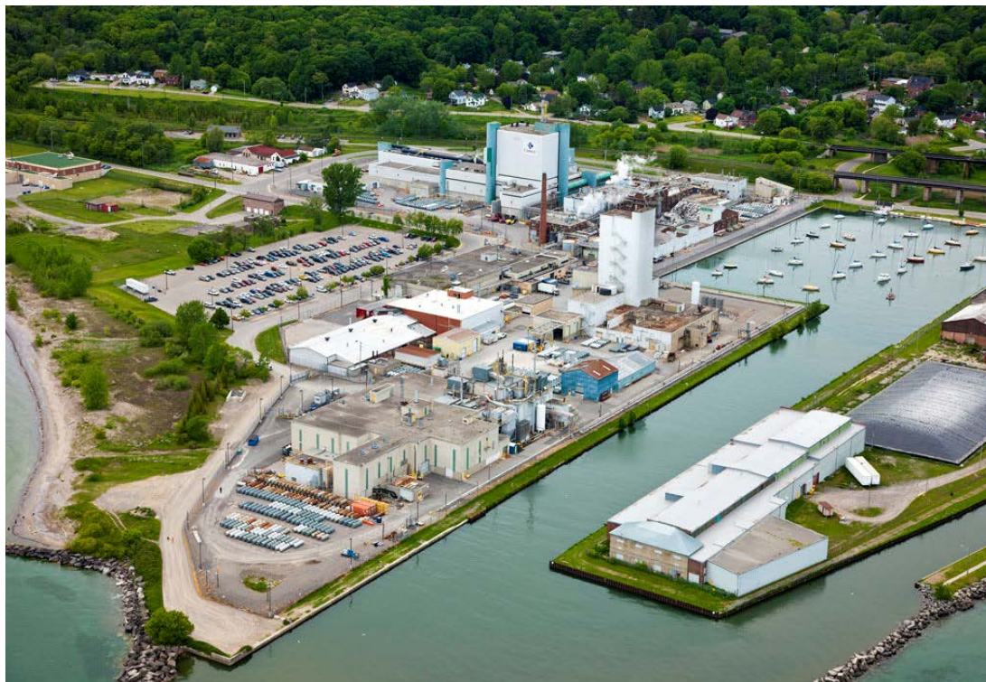
Figure 4-1: Port Hope Conversion Facility Site 1 (looking north)
